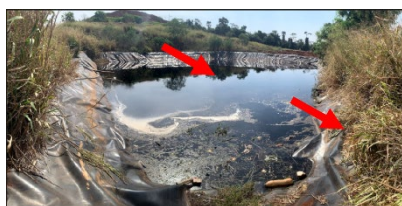
Figure 10. Leachate treatment pond
