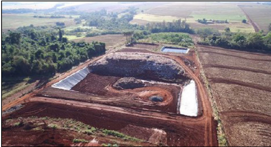
Figure 3. Existing ditch in the solid waste final disposal system
